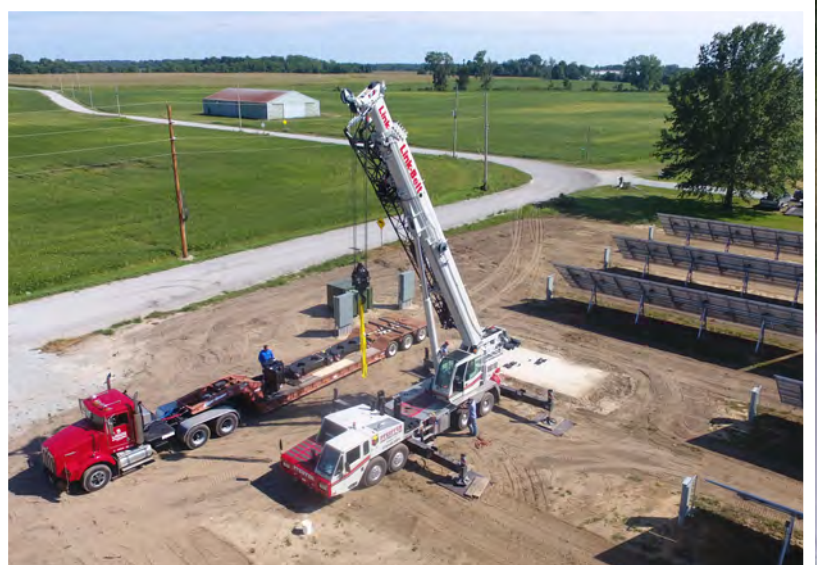
Crane cap setup for Megapack™ Battery Installation.
