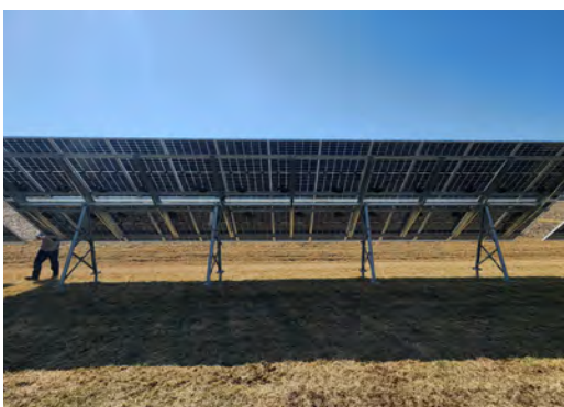
Rear View of cap array with Bifacial Panels
